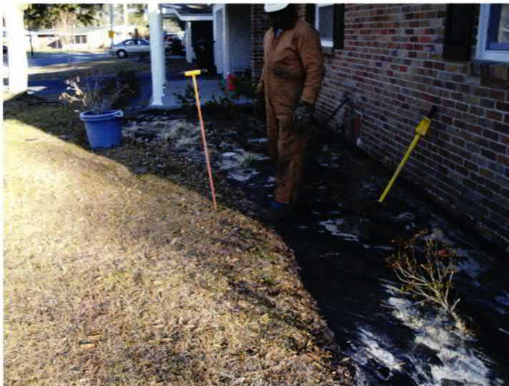
Picture 1: Location of UST 701Bluebell.
